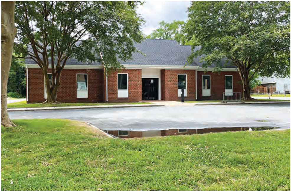
EASTERN SHORE POST/JIMMY SHOCKLEY The former Eastern Shore Public Library branch on Front Street in Accomac is being renovated into Accomack County offices.
